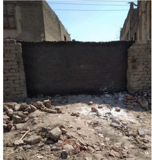
The newly reconstructed section of the site's surrounding security wall.
