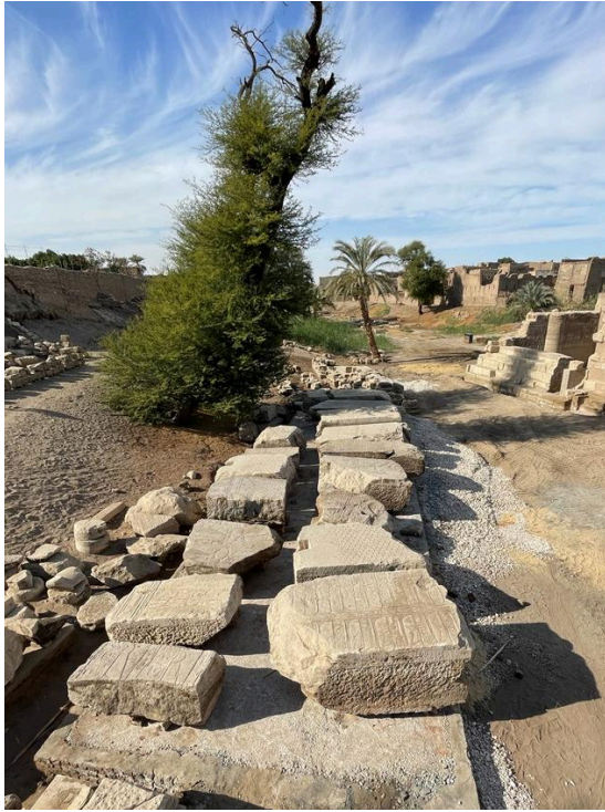
Cleaned, desalinated, and consolidated sandstone blocks resting on the new display platform that will prevent further damage from the elements.
