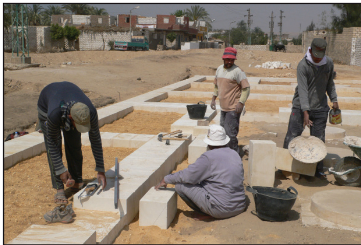
Team of builders from El-Till laying limestone blocks along part of the Great Aten Temple. March 2013. Photo by B. Kemp.
