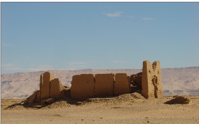
Fig. 1. One of the mud brick Roman period temples - this one has its pylon entrance largely intact.
